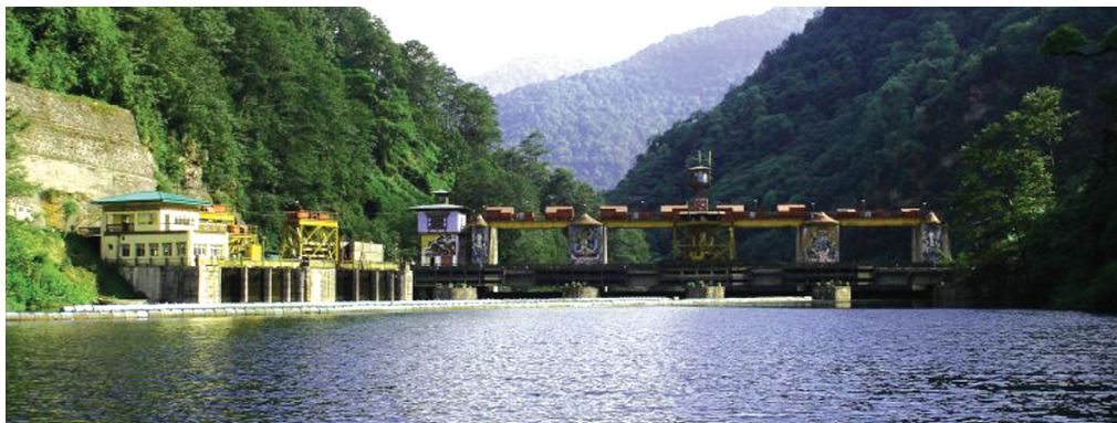
Figure 3 The 336MW Chhukha Hydropower Plant
