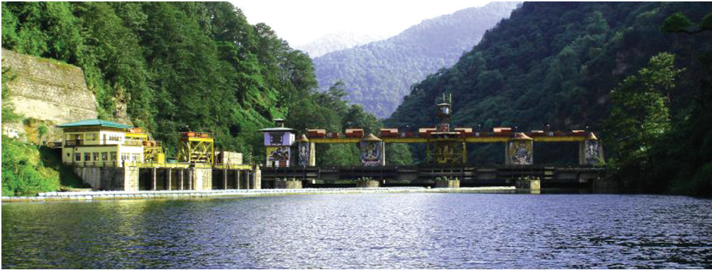
Figure 3 The 336MW Chukha Hydropower Plant
