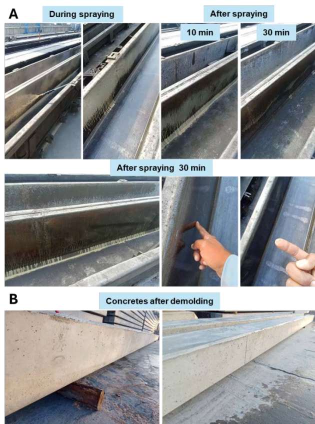
Figure 4 (A) Spray application onto steel molds for outdoor casting and (B) demolded concrete surfaces.
