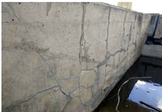
Figure 1 Cracking of the bridge foundation in Thailand.
