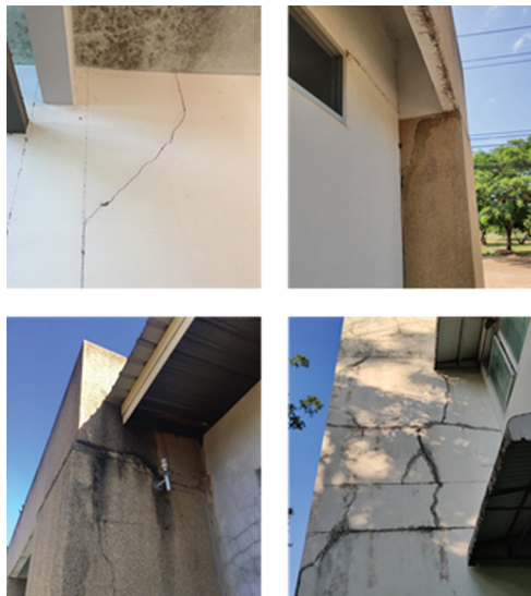
Figure 12 Structural cracks on KU CSC buildings due to settlement
