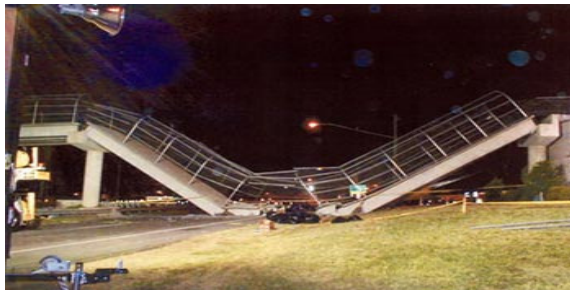
Figure 1 Bridge structure collapse due to corrosion failure [4]
