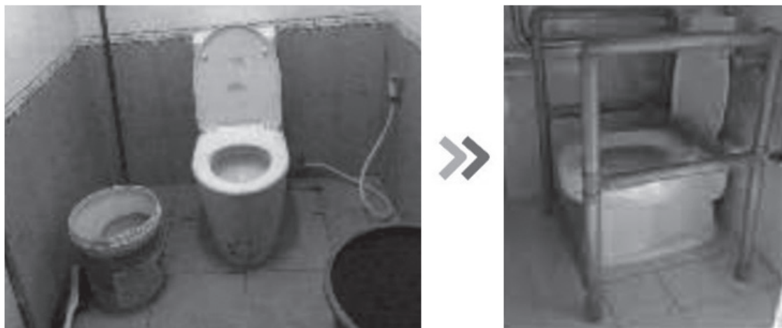
Figure 10: The toilet without a handrail of one of the samples (left) and an example use of the toilet rail innovation (right) (Sources: Photos taken by research team (Left), Faculty of Medicine Siriraj Hospital (Right))
