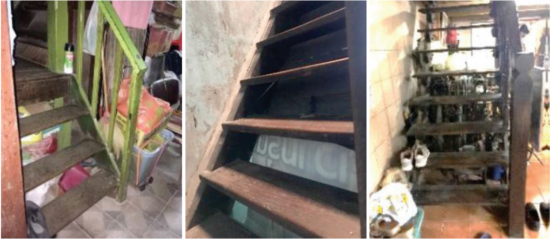
Figure 13. Inappropriate stairways found at the studied sites. (Sources: Photos taken by research team)
