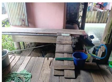
**High Hazards: Raised Wooden Stairs with No Handrails**
