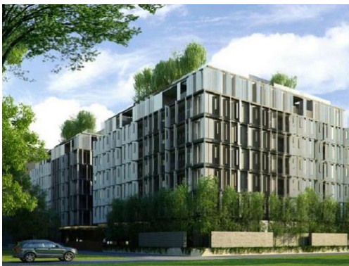
(a) Low-rise Condominium
