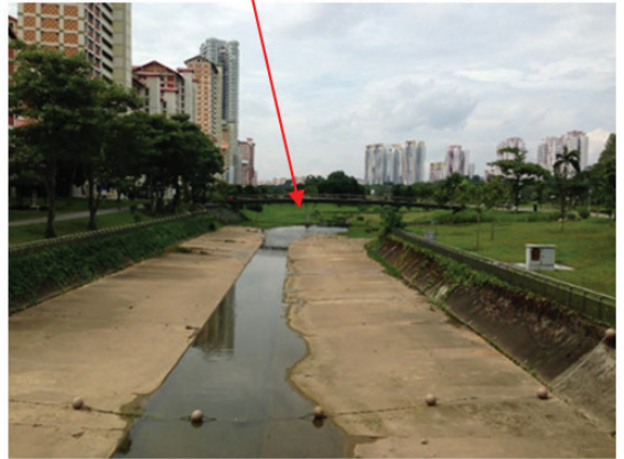
Figure 3: Bishan Park naturalized channel and floodplain (top, Google Earth Pro, imagery date 1 February 2019, Bishan Park, Singapore, 9 September 2019) and corresponding in situ photos of concrete channel draining the naturalized section of the park (lower right). The upstream park channel was concrete like this prior to 2012. Re-constructed (naturalized) river with mid-channel bars and functioning floodplain (lower left) (lower photos by the authors). HDB flats overlooking Bishan Park are observed in the background.
