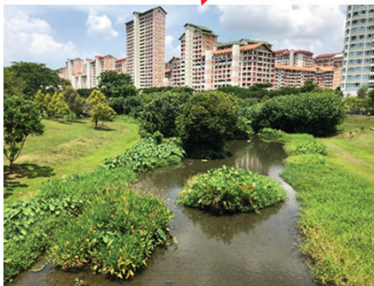
Figure 3: Bishan Park naturalized channel and floodplain (top, Google Earth Pro, imagery date 1 February 2019, Bishan Park, Singapore, 9 September 2019) and corresponding in situ photos of concrete channel draining the naturalized section of the park (lower right). The upstream park channel was concrete like this prior to 2012. Re-constructed (naturalized) river with mid-channel bars and functioning floodplain (lower left) (lower photos by the authors). HDB flats overlooking Bishan Park are observed in the background.
