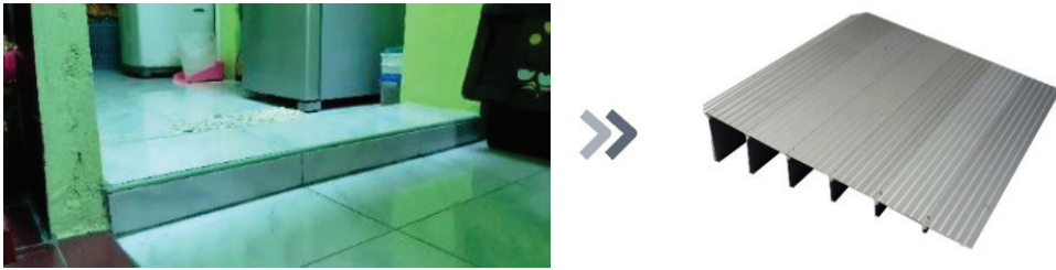
Figure 7: Uneven floor (left) and an example of a ramp (right) (Sources: Photos taken by research team (Left), Harmar Threshold Ramp - justwalkers.com (Right))
