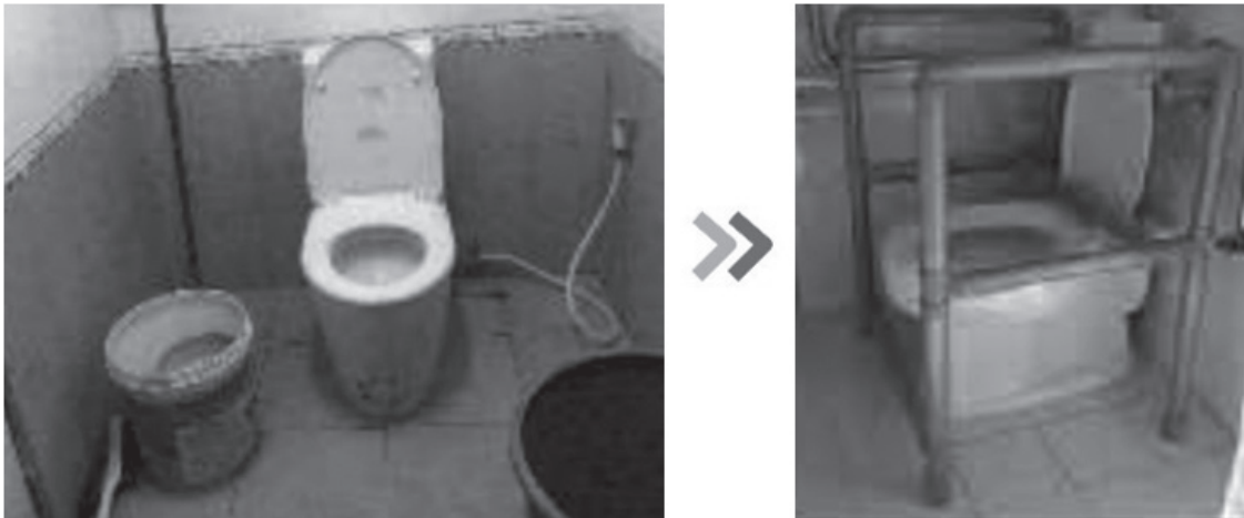
Figure 10: The toilet without a handrail of one of the samples (left) and an example use of the toilet rail innovation (right) (Sources: Photos taken by research team (Left), Faculty of Medicine Siriraj Hospital (Right))
