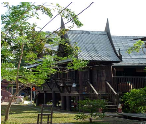
Figure 6: Thai house along Amphawa Canal
