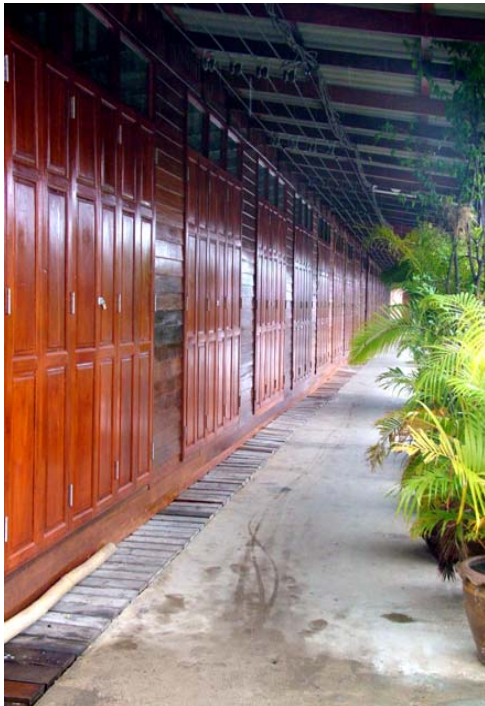
Figure 5: Folding doors or shutter in Amphawa row-houses
