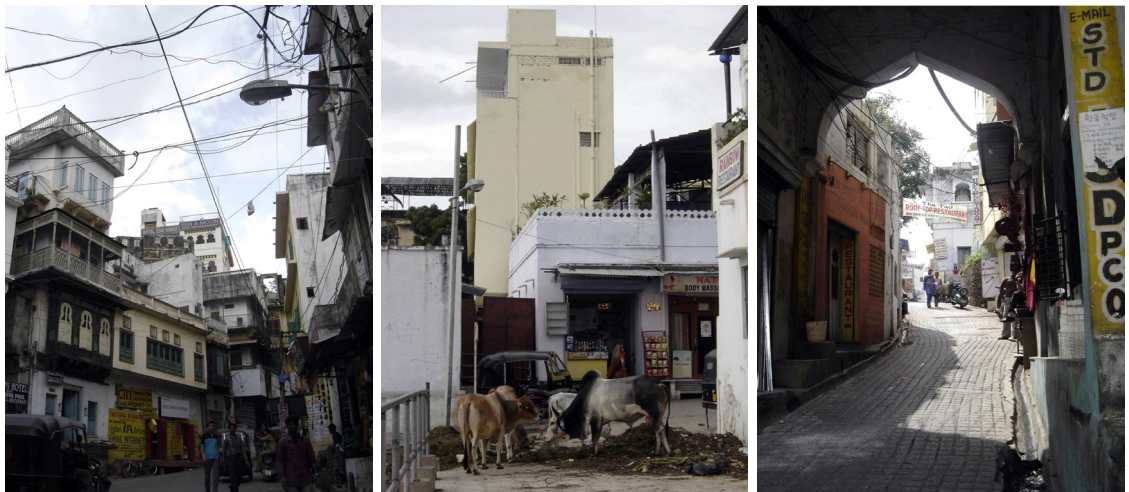
Figure 9: Visually Decaying - Hoardings, Graffiti, Electric Poles and Open Drains
