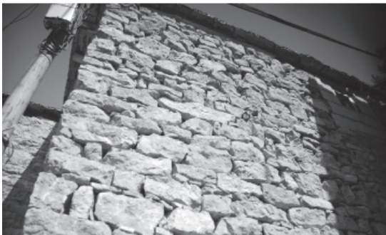
Figures 5: A wall without mortar.
