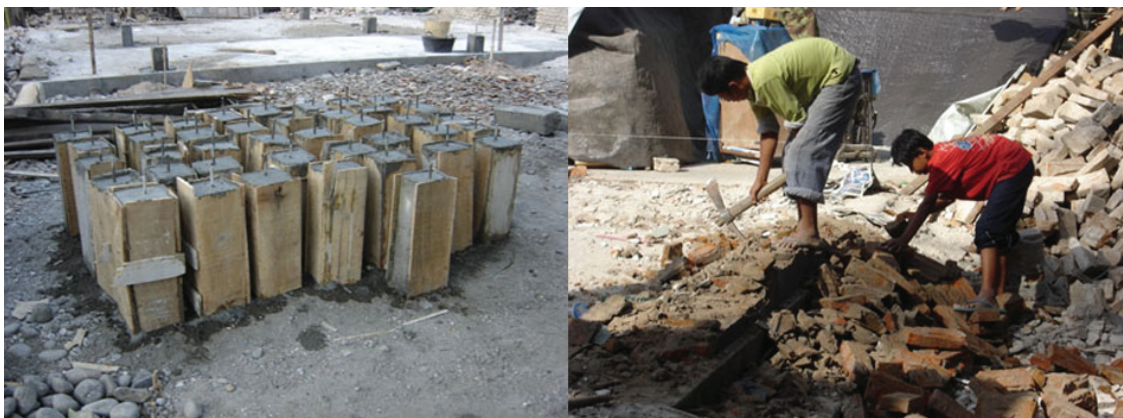
Figure 7: The concrete foundation (left); preparation of the place of foundation (right). Source: Prawoto, 2010.
