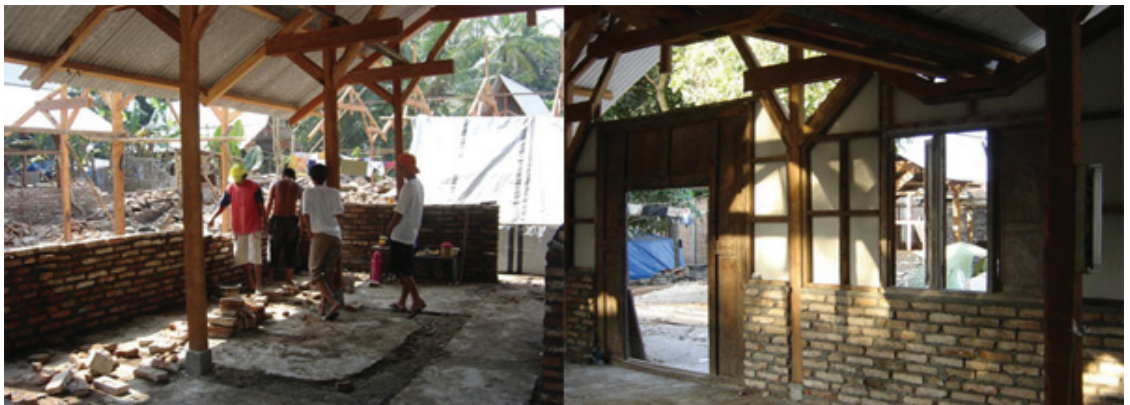
Figure 10: Making a brick wall (left); wooden frame clad with fiber cement board (right). Source: Prawoto, 2010.
