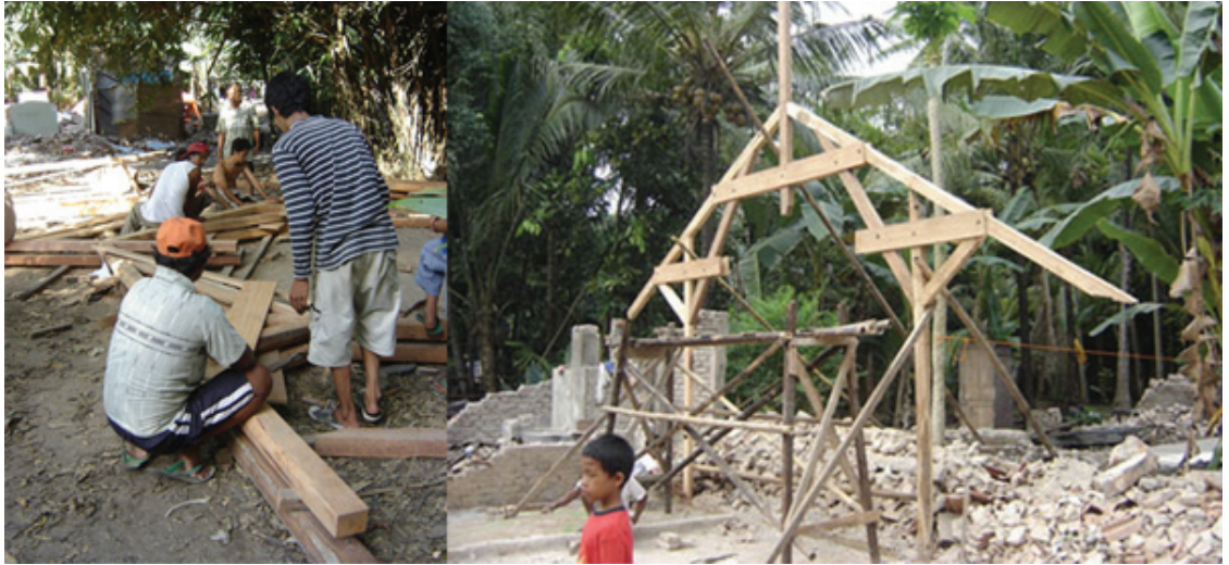
Figure 8: Preparing the coconut wood (left); the wood structural frame (right). Source: Prawoto, 2010.
