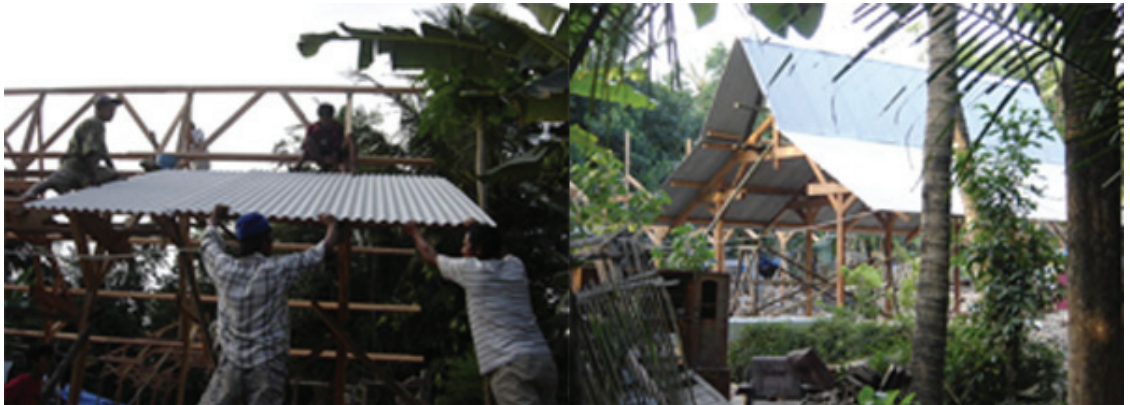
Figure 9: Installing the fiber cement roof (left); the finished roof cover (right). Source: Prawoto, 2010.
