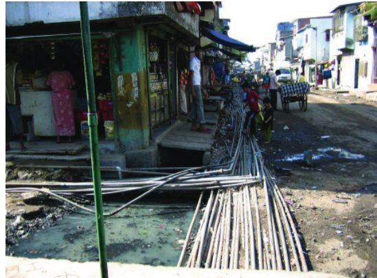
Figure 3: Consumer connections vulnerable to contamination
