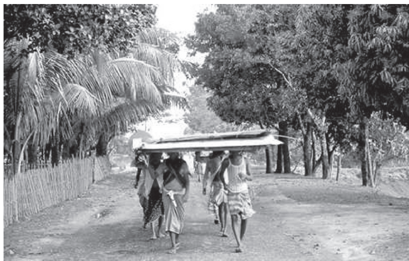
Photograph 1: House wall and roof sections are 'modular' and can be quickly disassembled and moved. (Source: Indra, 2000)
