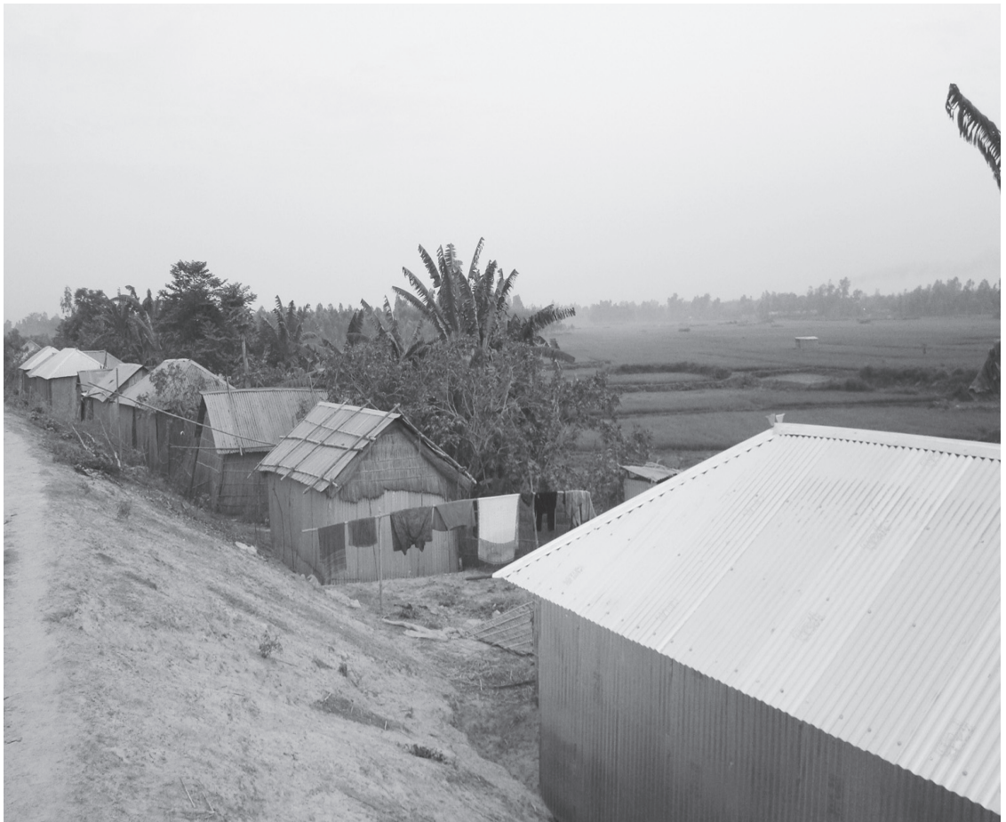
Photograph 6: Use of C.I. sheets as an enclosing and roofing material. (Photo by the author)
