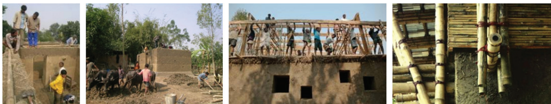
Figure 14: Construction Technique, and Bamboo joint Detail, Source: Anna Heringer, Open Architecture Network
