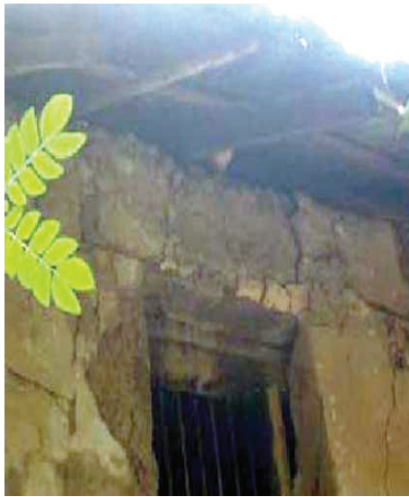
Figure 6: Cracking pattern of mud wall due to lateral load, Source : Rebeka Ahsan in Das et.al, 2007.
