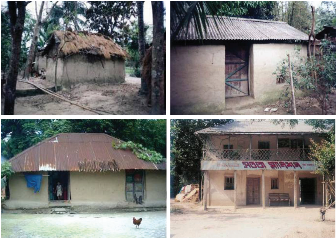
Figure 4: Typical building with thatch roof, tin roof, CI sheet roof supported by wooden purlins and a Two-storied mud house in Muktagacha, Mymensingh , Source : Asraful Alam 2006, Firoza Akter,2007 in Das et.al, 2007 .
