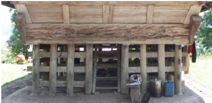
Figure 8: A system of beams into piles on flat stone
