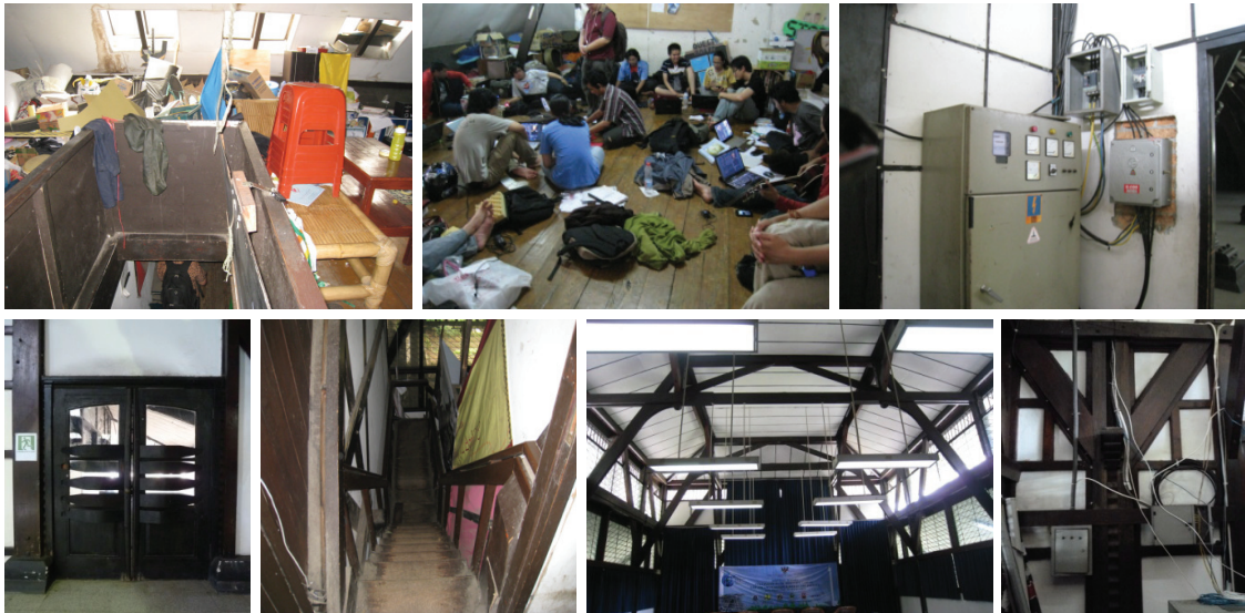
Figure 4: Combustible materials, inappropriate students' activities, insufficient emergency exit, lack of detection system and sprinkler, insufficient exit signage and lack of maintenance of electrical installation/wiring in the Assembly Halls Source: L. Tambunan (2013)
