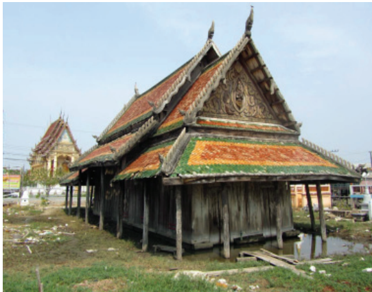
Figure 8: Wooden structures of the ordination hall at Wat Srang Sok, Samut Prakan
