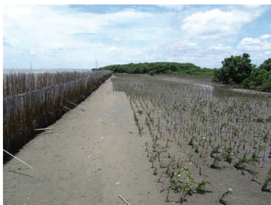
Figure 2: bamboo barriers as offshore breakwaters on the coast of Samut Sakon Province (left) and mangroves were planted behind the barriers on the coast of Samut Prakan Province (right)
