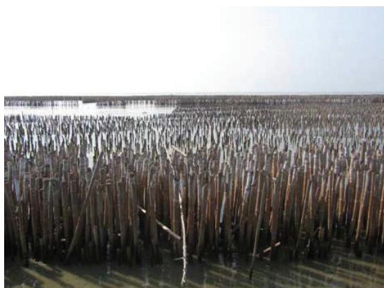
Figure 2: bamboo barriers as offshore breakwaters on the coast of Samut Sakon Province (left) and mangroves were planted behind the barriers on the coast of Samut Prakan Province (right)
