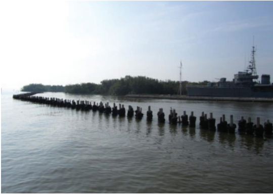
Figure 3: pre-stressed concrete poles and outer tyres built offshore in front of the Chulachomklao Fortress, Samut Prakan Province
