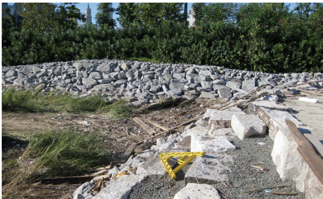
Figure 12: Destruction and debris in the salt marsh following Hurricane Sandy.
