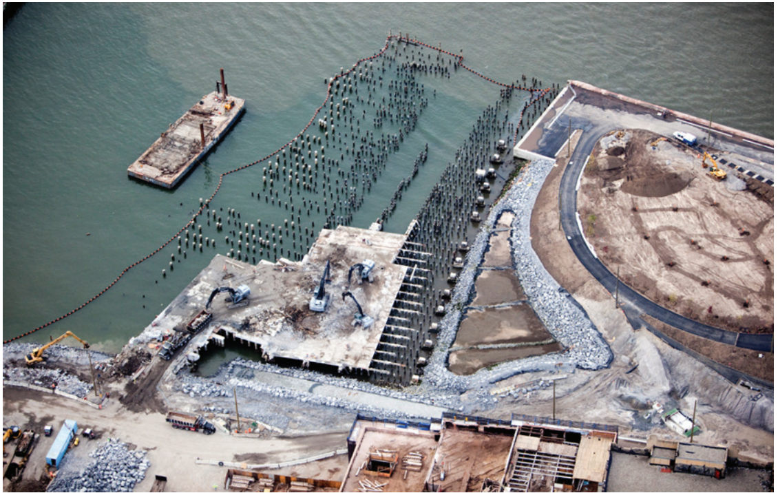
Figure 8: Aerial photo of the salt marsh under construction. Voids in the pile field trace the paths of two underwater tunnels serving the A and C subway trains
