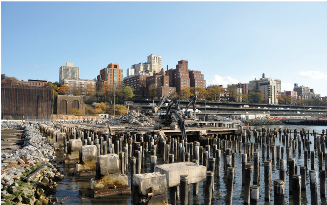
Figure 7: The concrete pier decking is removed, exposing the pile field beneath.
