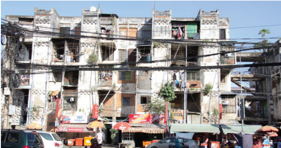
Figure 6: West elevation of block A of White Building. Courtesy of Pen Sereypagna.
