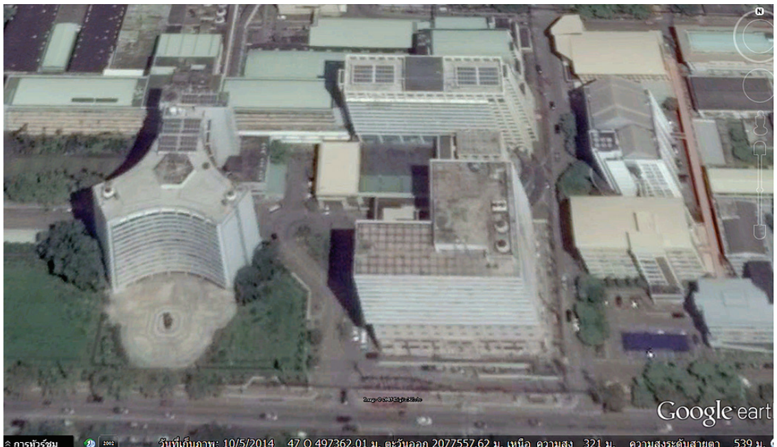
Figure 4: Building Characteristics from Google Street View at Maharaj Hospital, Chiang Mai City
