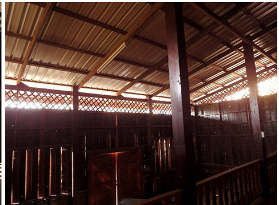
Figures 36: Kor-Song, the wall vents with cross bracing wood.
