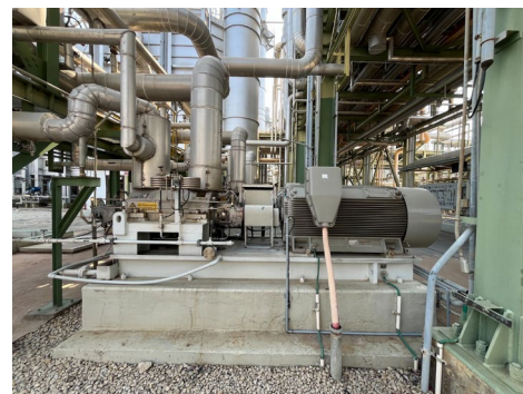
Figure 1 Boiler Feed Water Pump (BFP)
