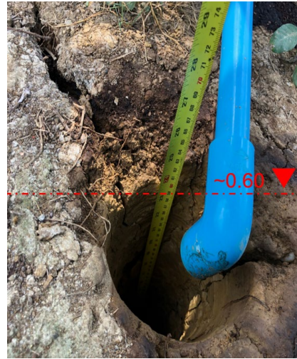
Figure 12. The remaining depth of the hole full with KOH flakes and water was about 0.60m.
