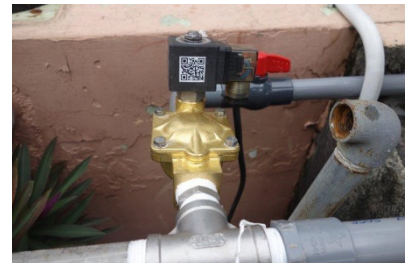
Figure 5 Soil Moisture Sensor, EC (pH) Sensor and Solenoid water valve installation
