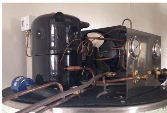
Fig. 4. A 5-kW air-to-water heat pump.
