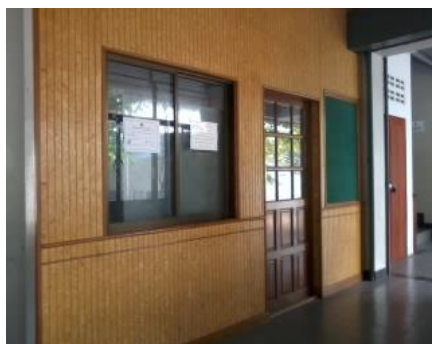
Fig. 26 Using oriented strand boards from rice straw and maize husk to install with building wall
