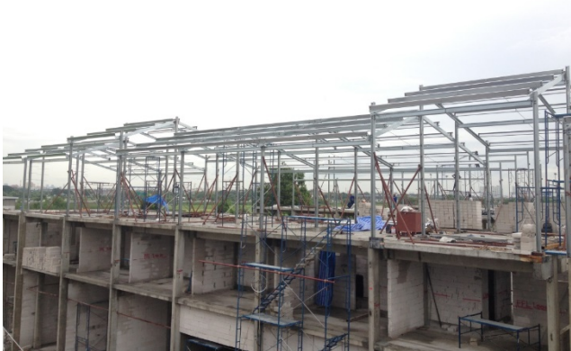
Figure 1 Use of light gauge steel and block wall for real estate industry in Thailand
