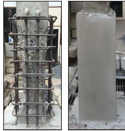
Figure 3 Repairing of damaged column
