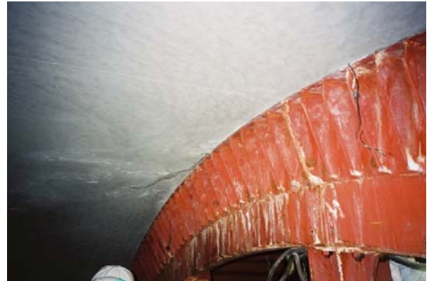
Figure 8 Self-compacting casted into an arch crown of a tunnel
