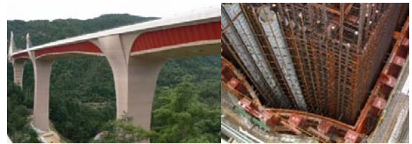
Figure 7 High pier of bridge and confined zone of reinforcing bars
