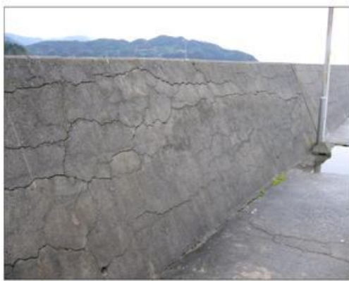
(1) Breakwater at seaside. Map cracks showing some preferred horizontal orientation because the expansion in longitude direction is restricted. Maximum opening of cracks reaches several cm partially because of almost no reinforcement.
