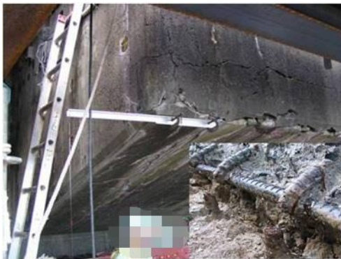
(3) Crossbeam of road bridge. Maximum opening reached 10 mm and reinforcement breakages were observed.
