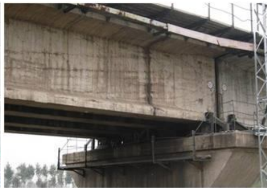
(4) Prestressed concrete girder. Cracks along reinforcement are characteristic appearances for this kind of prestressed structure.
