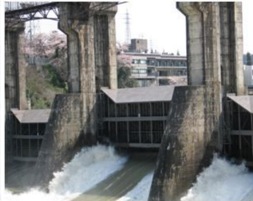
(2) Dam gate. In the case of dam structures, only small expansion becomes problem to affect the movement of gates.
