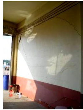
(a) Cracks on a wall
