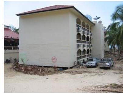
(b) Three-stories building was damaged in secondary members only
