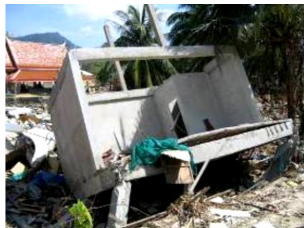
(a) Joint failure
