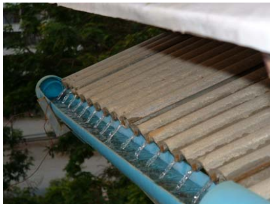
Figure 2 Flow of water through the grooves of the cement tiles of the roof pond house
