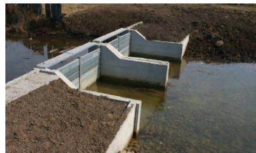
Figure 7 Weir (Stop Log) [15]
