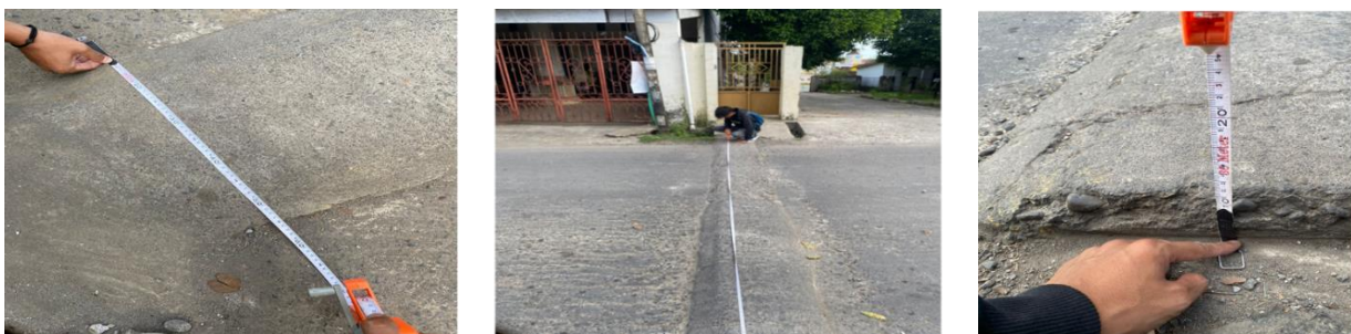
Figure 1 Speed bump measurement (width, length, and height)
