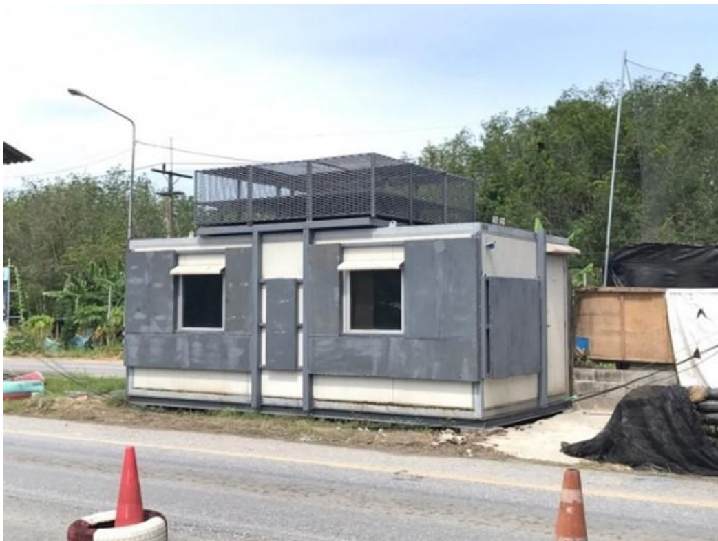
Figure 12 Buildings installed the bulletproof panels from the study.
