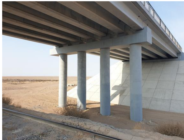
Figure 2 View of pier No. 3 and the embankment cone of abutment No. 4.
