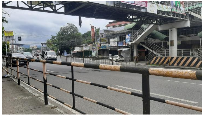
Figure 4 Barriers at MSU-IIT Badelles Overpass
