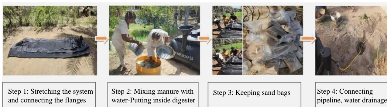
Figure 6 Construction of a HomeBiogas system
