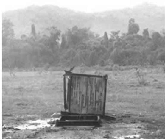
(c) Steel structure after blasting demolition
