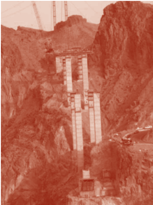
Figure 11 Foreland bridge piers construction.
