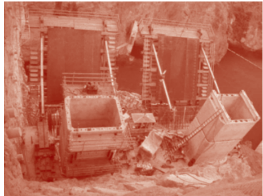
Figure 12 RC arch rib construction.
