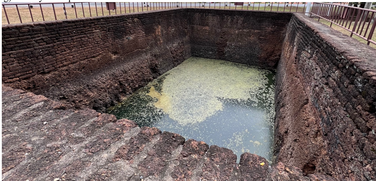
Figure 2 Bo Sam Saen located at a laterite mound in Wat Awat Yai, Aranyika region of Kamphaeng Phet Historical Park, showing walls of a pond built from laterite at Nong Pling Sub-District.
