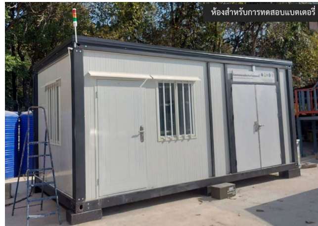
Figure 9: External of test chamber
