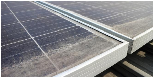
Figure 6: Examples of potential dust on the solar panels [23]
