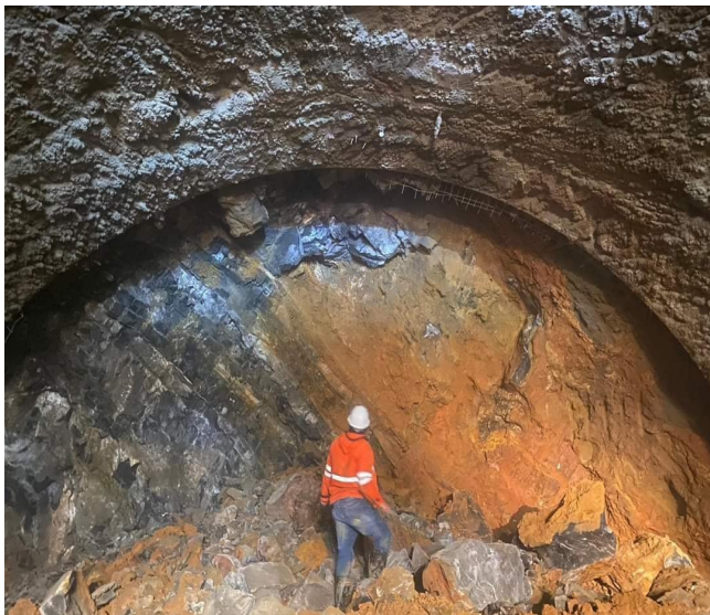
Figure 18 Tunnel face after blasting at Sta. 131+720.4 using the proposed approach
