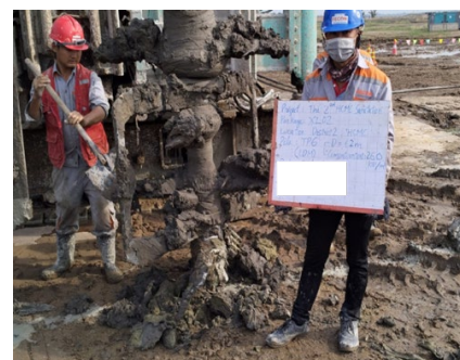
(a) 0.5 m/min (down), 1.1 m/min (up), rotation 17 rpm
